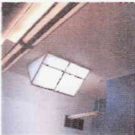
+ ENLARGE The reflective concrete ceiling, along with lightshelves and sunlight shafts, reduce energy use and air conditioning load.
