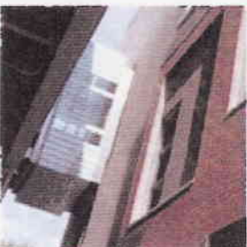
+ ENLARGE With Chicago's elevated train running less than 10 feet from the center, concrete helps reduce noise transmission.
