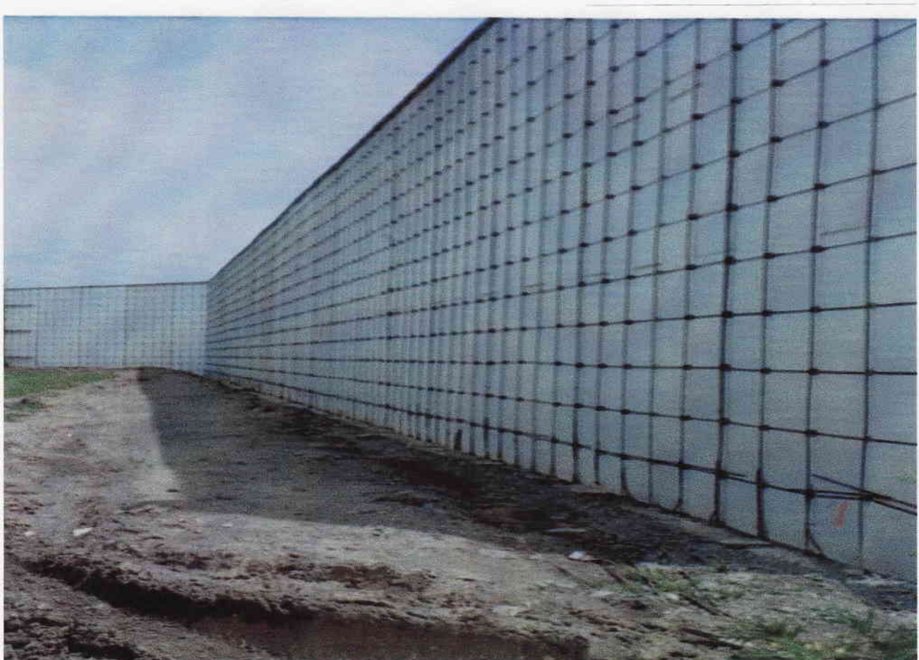
Wall ready for Shotcrete
