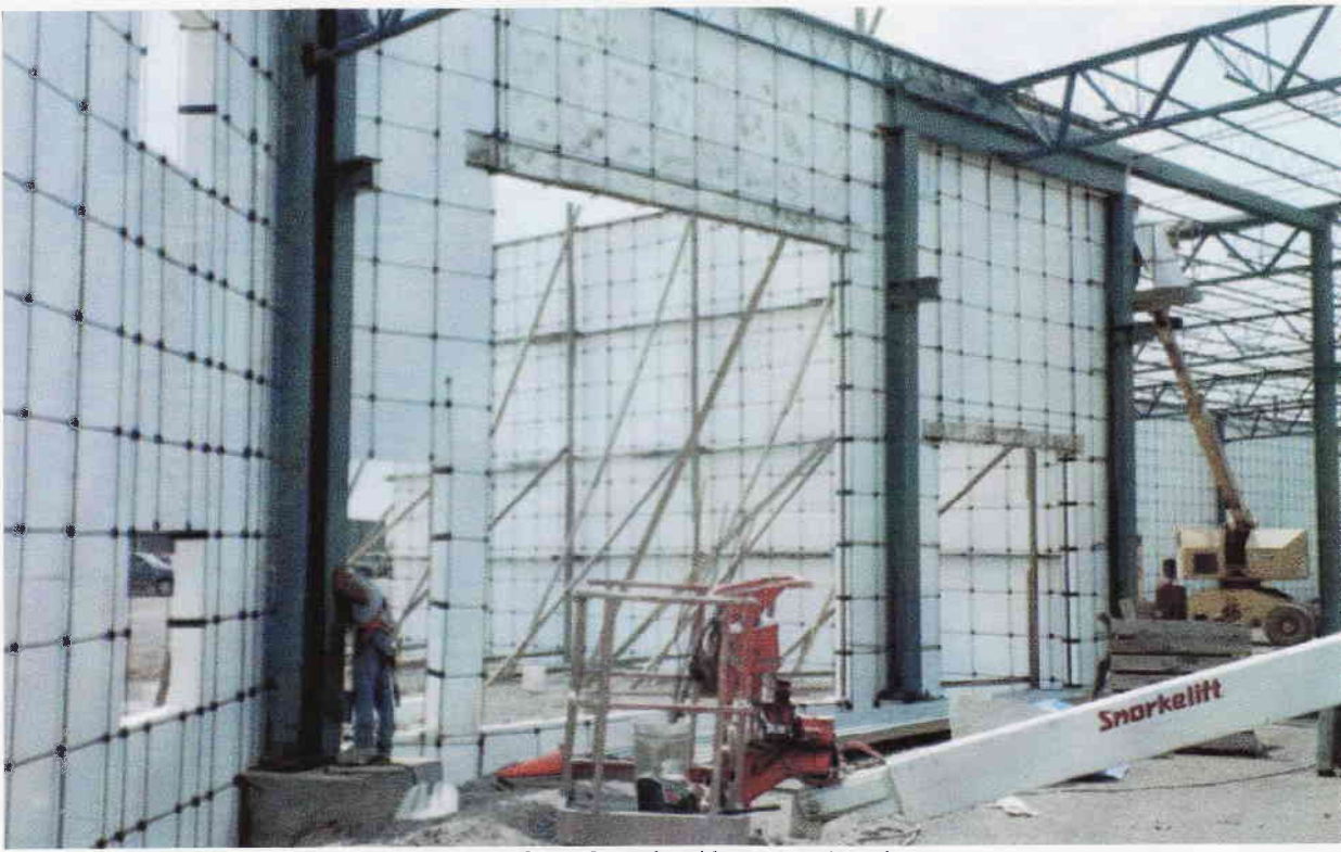
Interface of panels with structural steel
