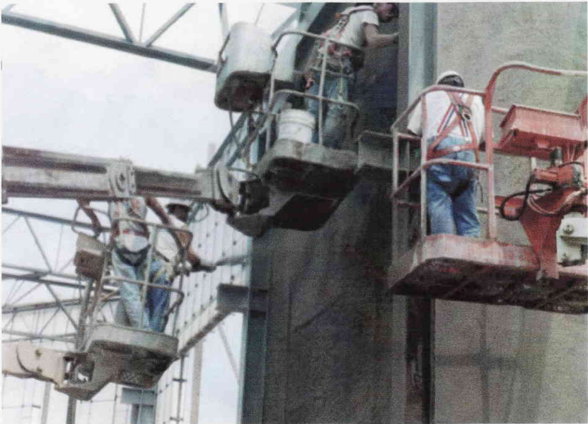
Shotcreting, screeding and finishing the walls
