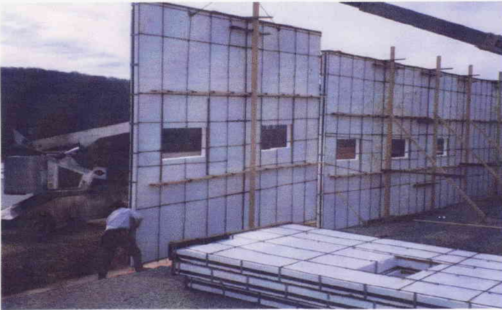
Setting panels on footers
