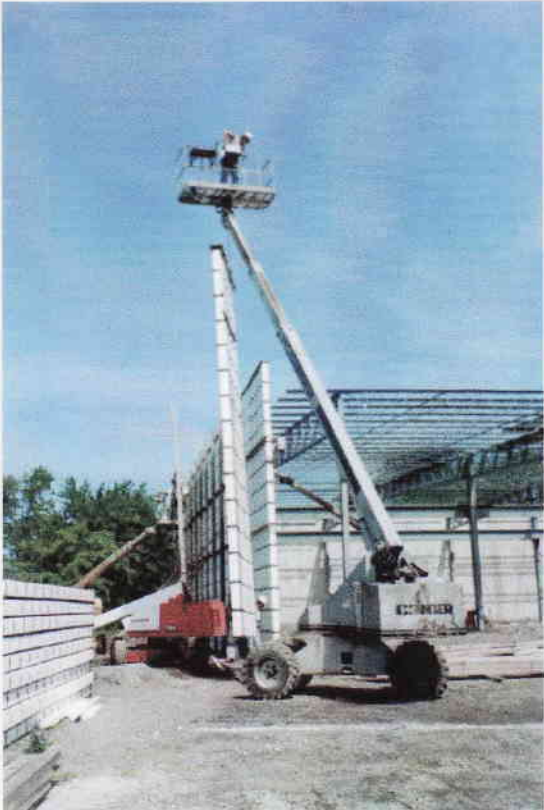
Erection of lightweight wall panels
