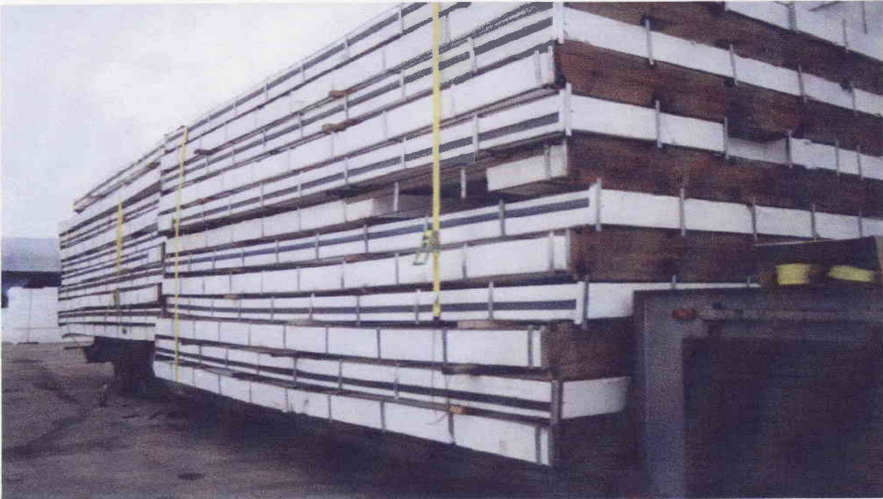
Load of wall panels delivered to jobsite
